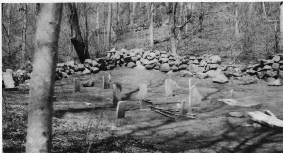
The Rathbun Cemetery as it looked just after it was cleared and before the gravestones and rock walls were repaired.
